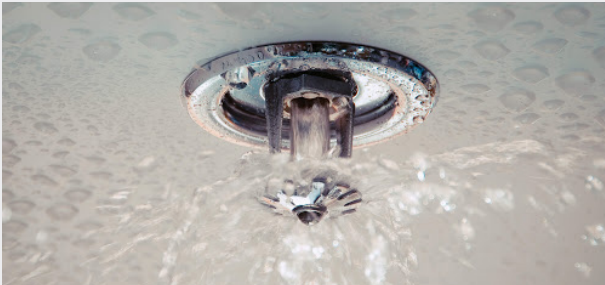
Discharge might occur if a sprinkler head is accidentally overheated or damaged
